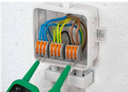
Testing the wired connectors.
