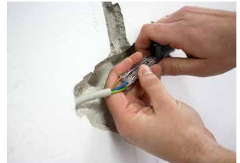
Connect the cable using the cable repair kit.
