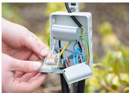
Connecting a bollard light
