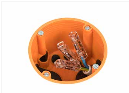
Extending short wires.
